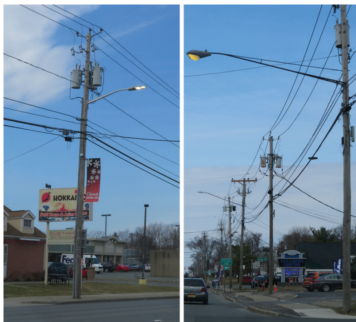
Lighting along Central Avenue (Rt. 5). Left: LED lighting in the City of Albany, NY. Right: Traditional cobra head lighting in the Town of Colonie, NY. Photos by Planning4Places, LLC
