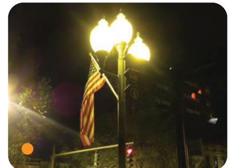
Historic pole-mounted lighting: Public decorative triple post top (unshielded, 360 degree light)
