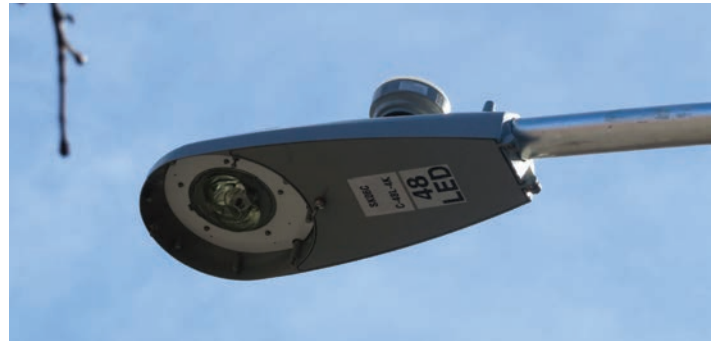
Example: Smart hardware visibly attached (Schenectady, NY) Photo by Planning4Places, LLC
